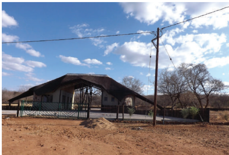
Figure 3: MmaMotshwane Gate House (photograph by Phenyio Thebe 2012)
