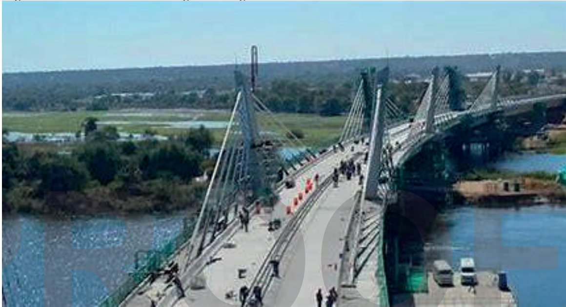
Figure 3: Picture of the Kazungula Bridge 10
