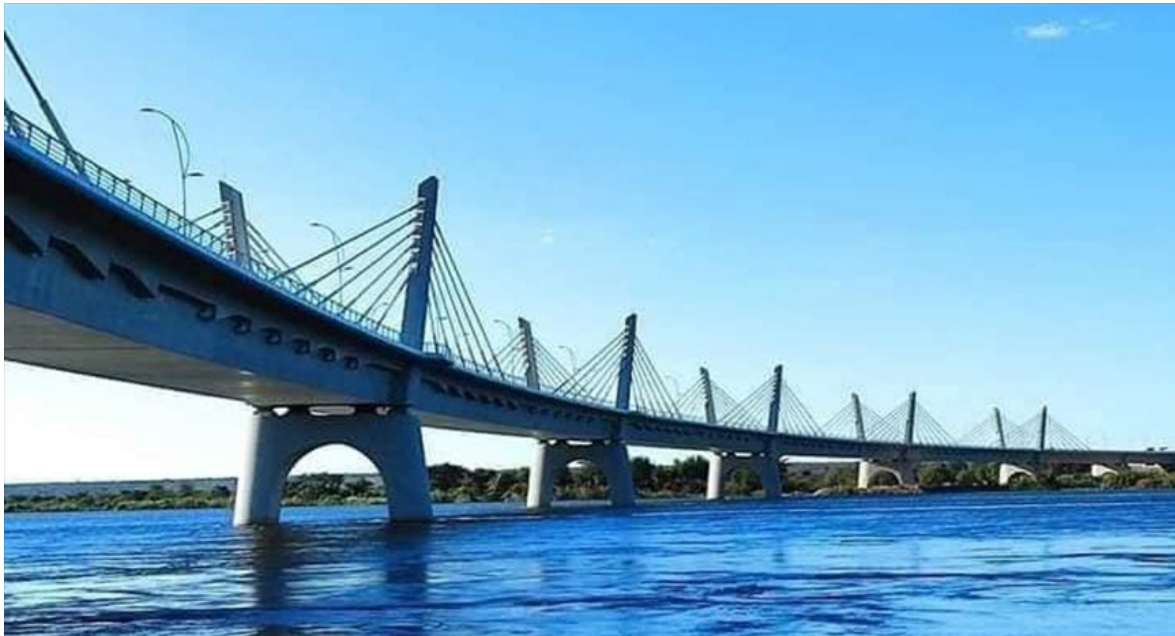
Figure 1: The Kazungula Bridge after completion. 1
